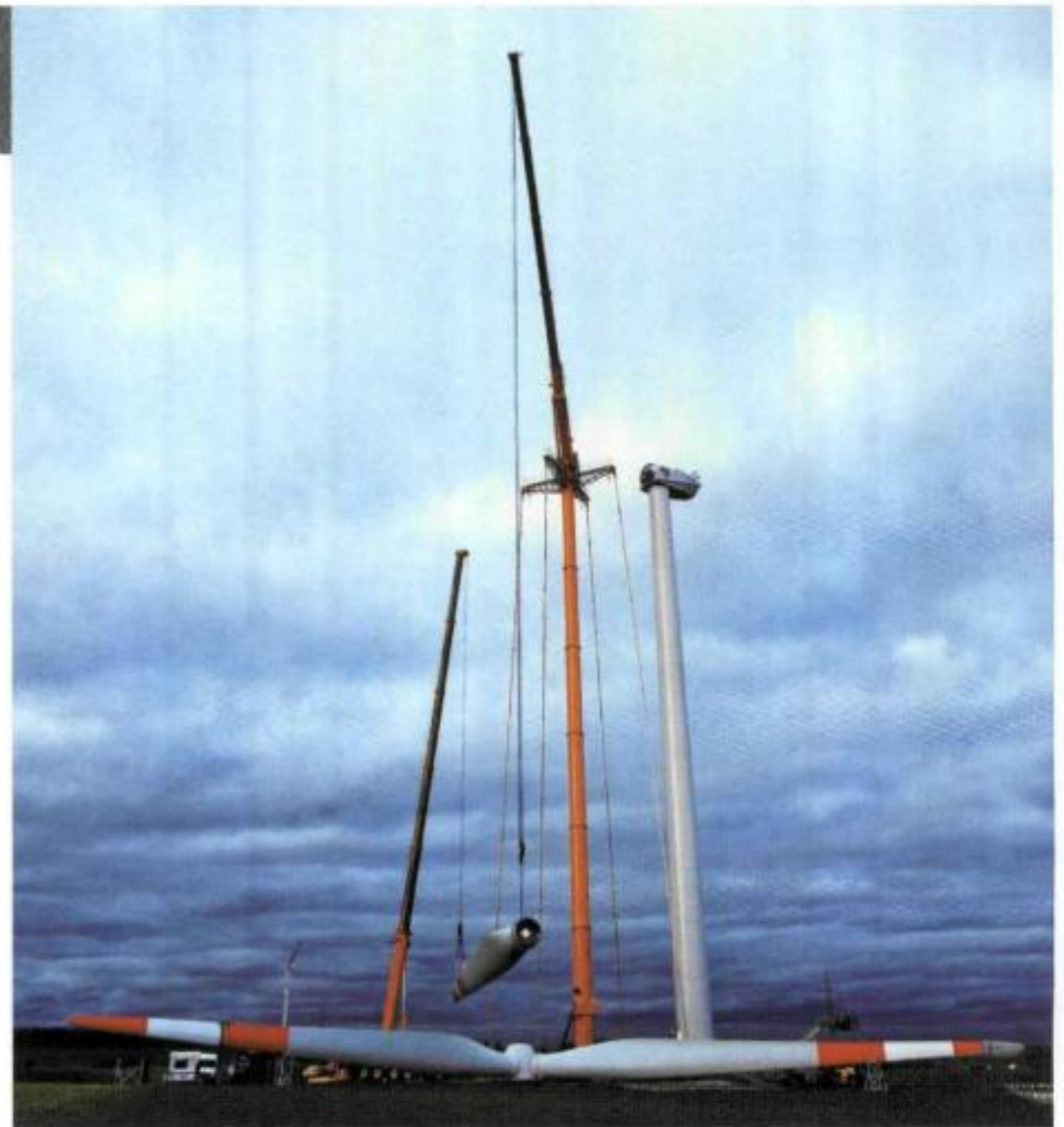
Vanguard's new R70-million crane can lift 100 t to heights of more than 100 m.
